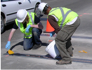
Pouring Grout into Slot
