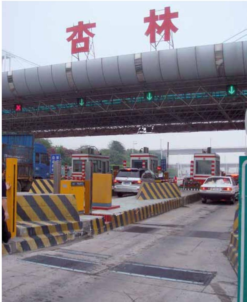
IRD's PAT Bending Plates installed in toll lanes at a toll plaza in Fujian province in China. IRD's WIM@Toll system is installed at this site before vehicles cross the Xinglin bridge in Xiamen
