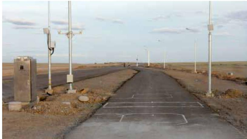
**IRD's WIM@Toll system installed in Mongolia using IRD's slow speed WIM scales. IRD's system also includes automatic vehicle identification (AVI) using RFID transponders and readers**
