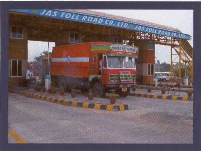
IRD iTOLL System installed for JAS Toll Road Co. Ltd. near Bangalore, India.
