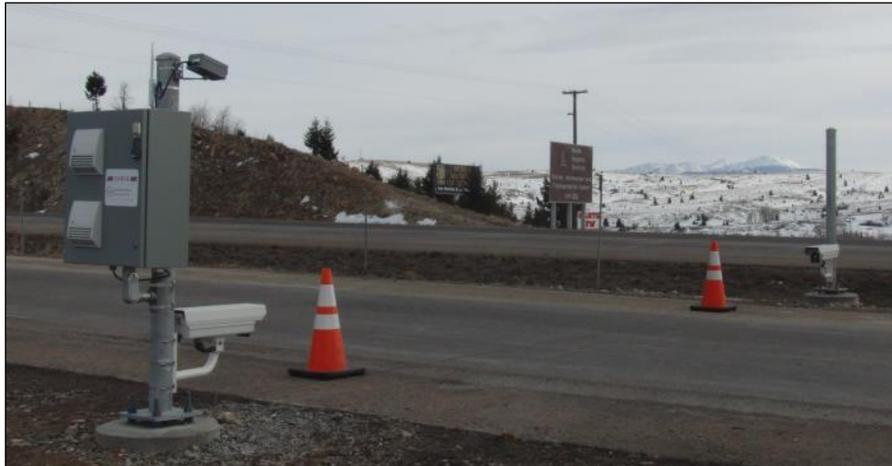
**Figure 5 – Infrared Cameras and Thermal Imaging System Enclosure**
