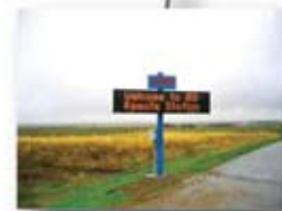
VMS-VARIABLE MESSAGE SIGN
