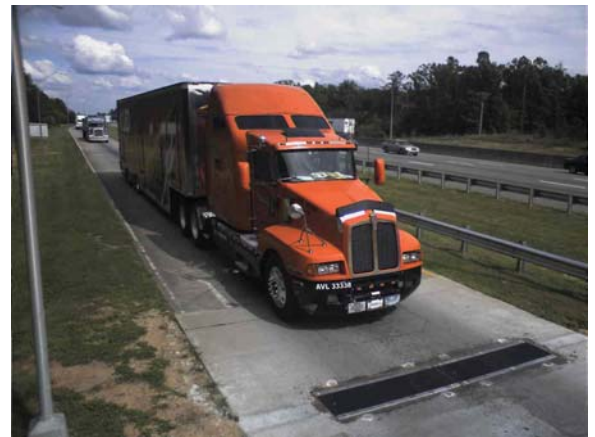
Truck passing through a Virtual Weigh Station using IRD-PAT Bending Plate™ WIM Scales
