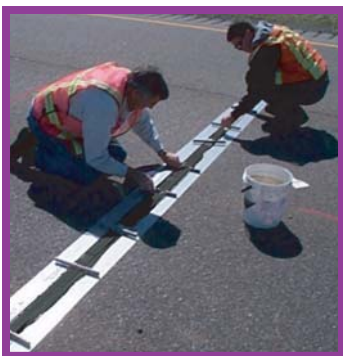
Inserting Sensor into Slot
