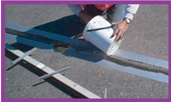
Pouring Grout into Slot
