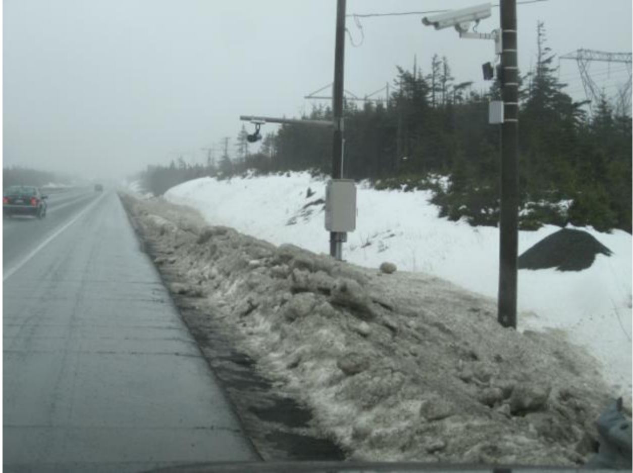
Figure 10 – Virtual Weigh Station with License Plate Reader and Side View Camera, Newfoundland
